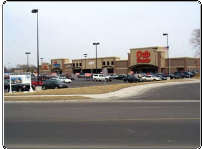
Construction of a new Cub Foods store was a key element in the Lyndale Green redevelopment project in Bloomington, MN.
