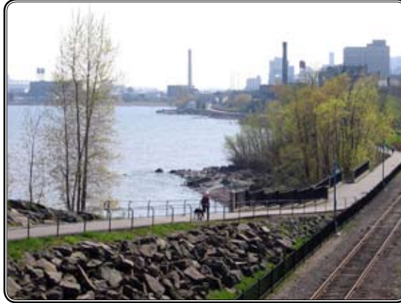
MSA is working with the City of Duluth, MN to prevent sanitary sewer overflows caused by the heavy clay soils and aging infrastructure.
